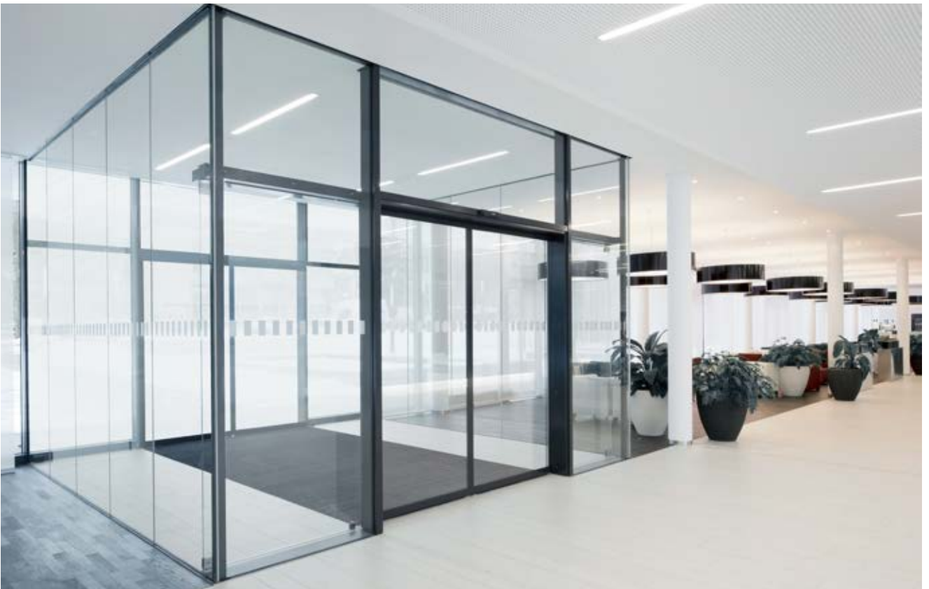
Slimdrive SL NT with vestibule, Augustinum, Stuttgart, Germany (photo: Dirk Wilhelmy)
