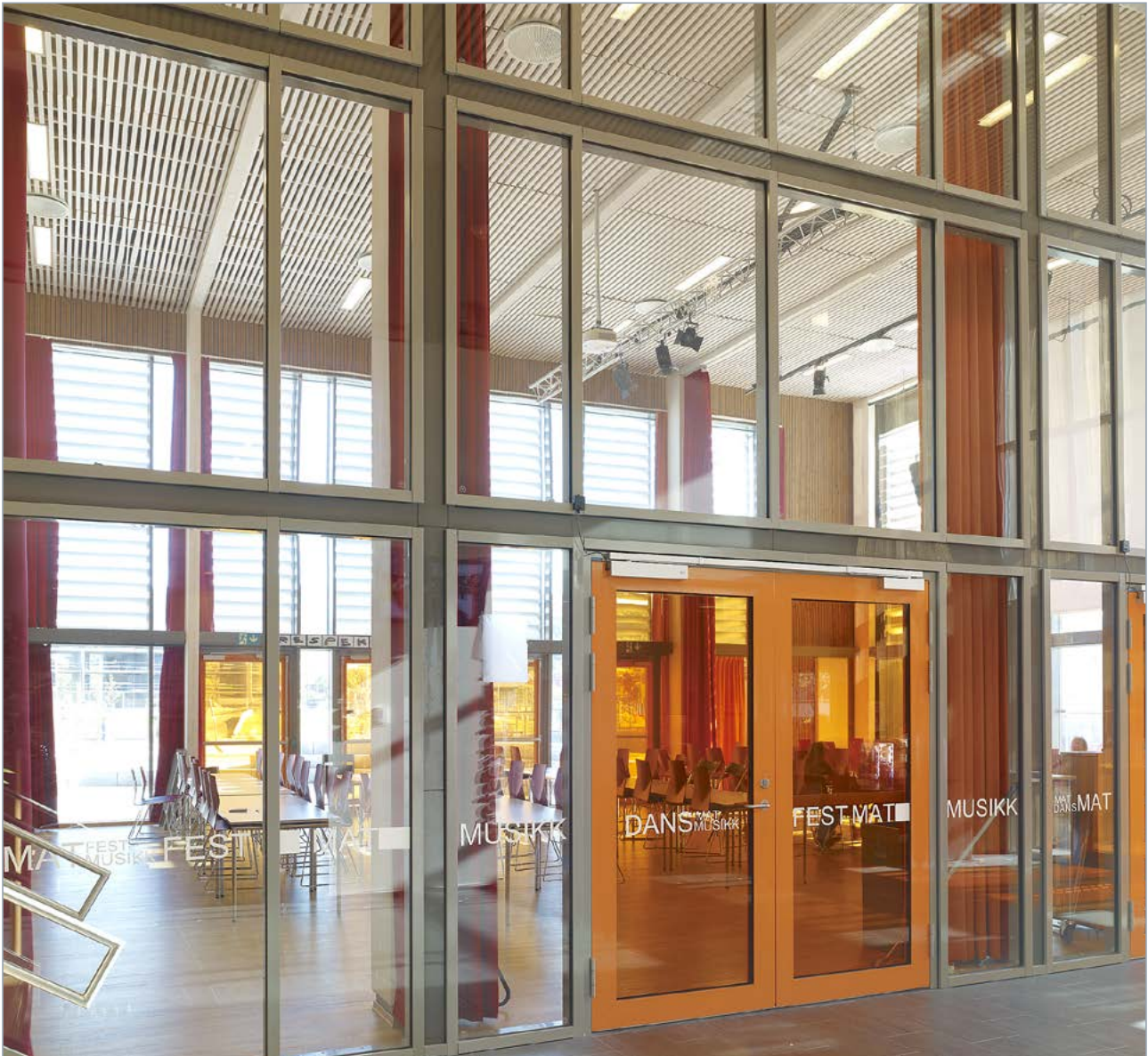
Ranheim School in Norway uses Sapa Facade 4150, meeting fire protection class EI30, for interior elements.
